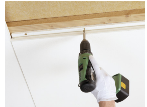
Master F is installed by screw fixing
